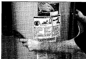
ROTATE INWARD UNTIL V-GROOVE IS FACING DOWN
