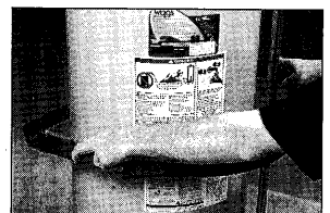
ROTATE INWARD UNTIL V-GROOVE IS FACING DOWN
