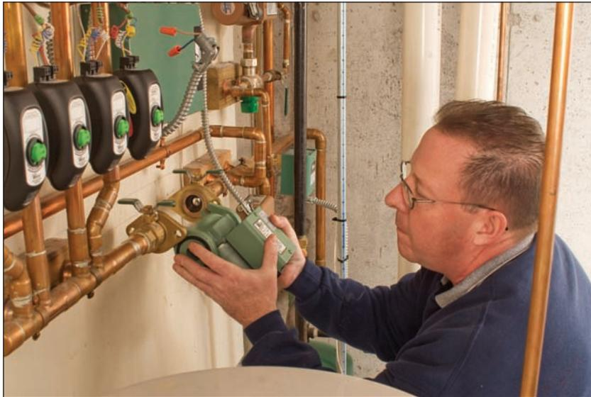
Harry Grattage, technician for Riley Plumbing, installs a variable speed circulator.
