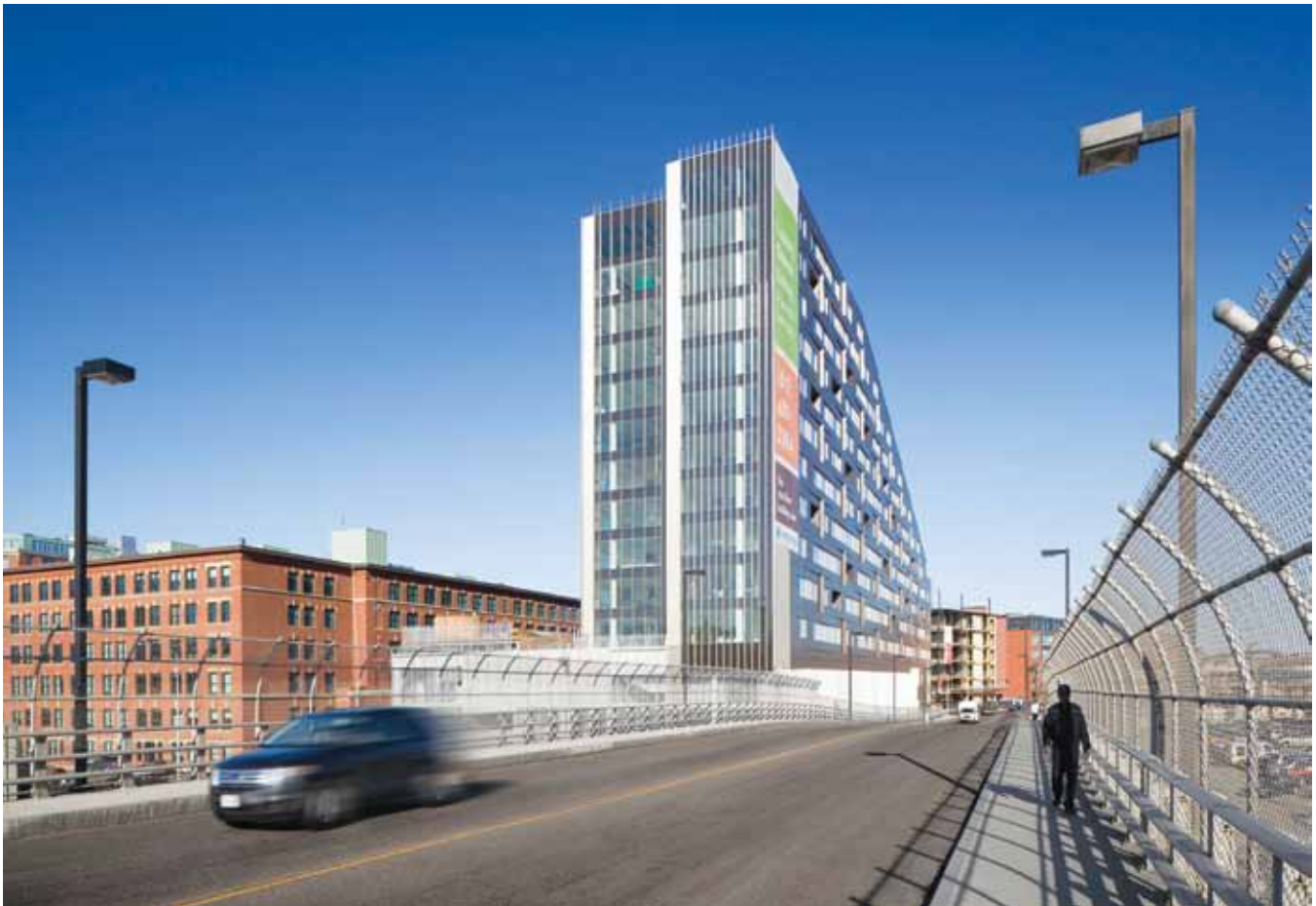
Macallen Building Condominiums, Boston; architect: Burt Hill, Office dA; photo by John Horner Photography 2008
